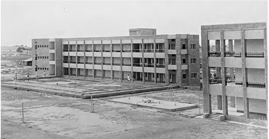
The rising structures (AKJCB).
