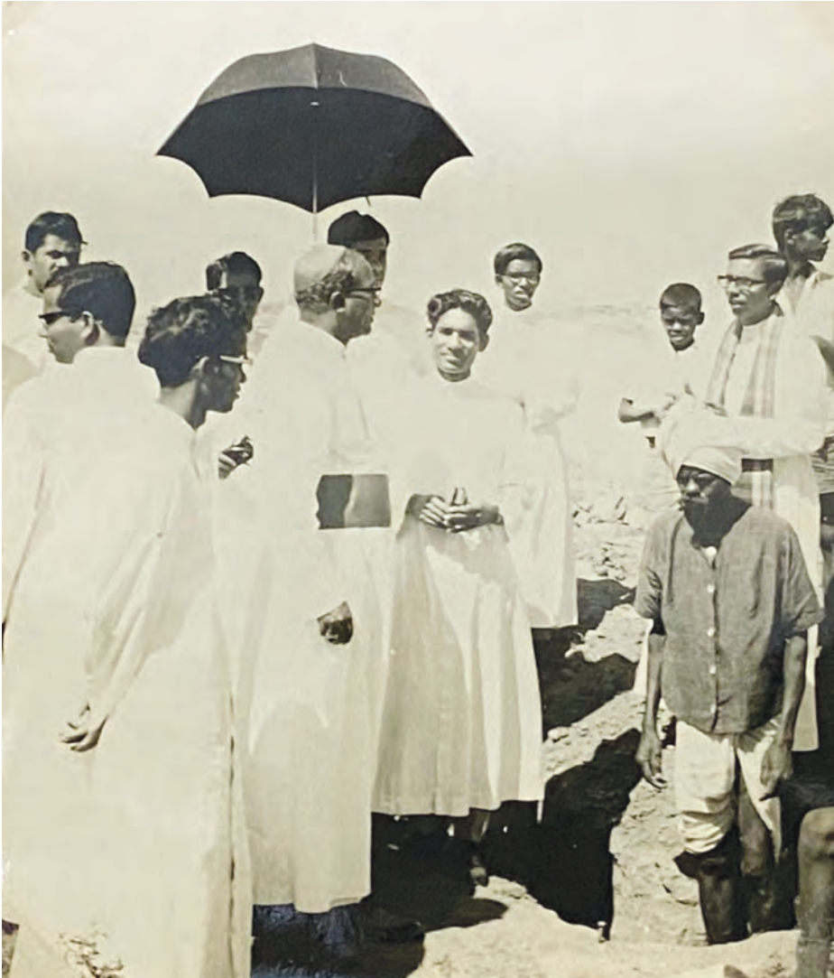
Archbishop Packiam Arockiaswamy, Archbishop of Bangalore (1971-1986) visiting the site of a building under construction (AKJCB).
