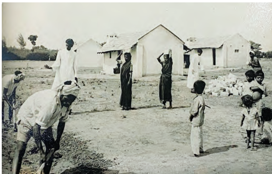
Digging the foundation for a new house (AKJCB).
