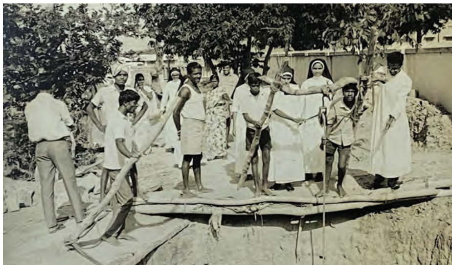
Digging a well to provide water for the villagers in collaboration with the Sisters of St. Anne, Bangalore (AKJCB).
