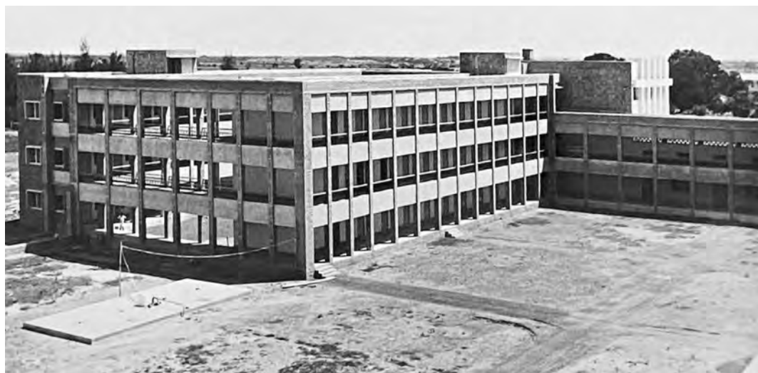
The rising structures (AKJCB).
