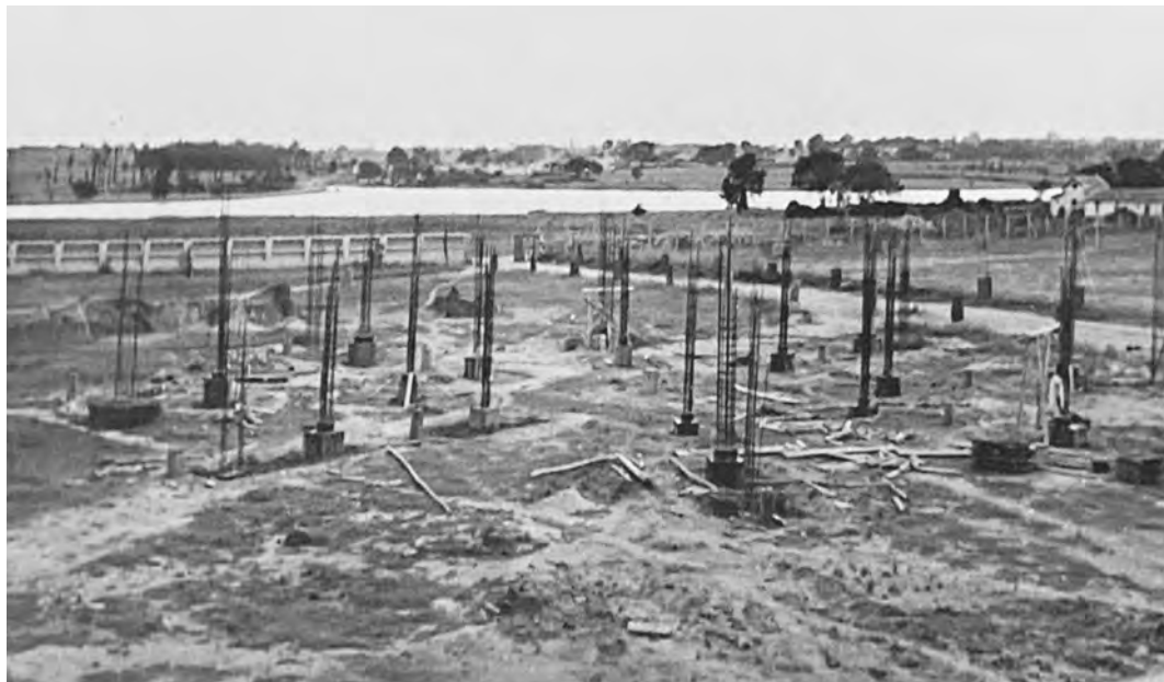
Kristu Jyoti College: Construction in its earliest phase (AKJCB).
