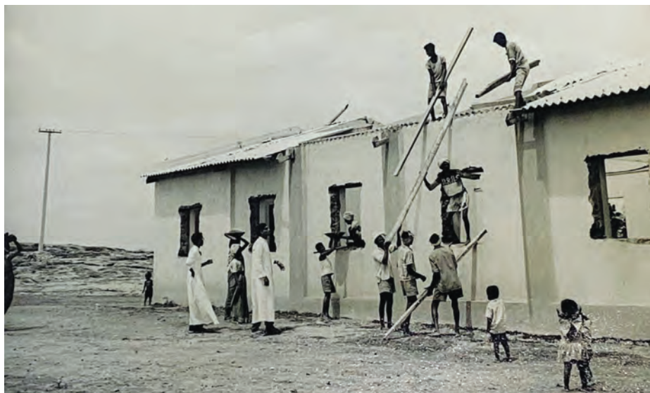
Students of Kristu Jyoti supervise the roofing of the new houses built by S.S.G. (AKJCB).
