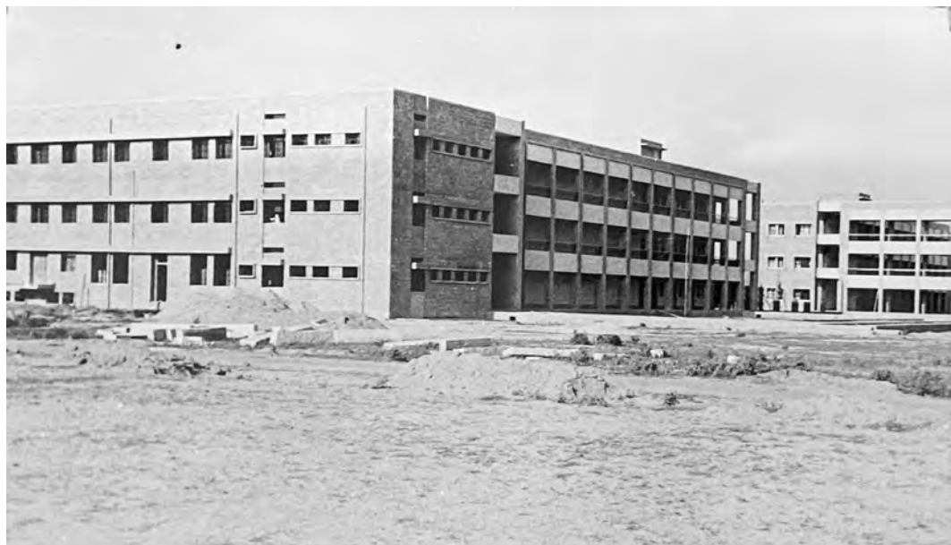
The rising structures (AKJCB).
