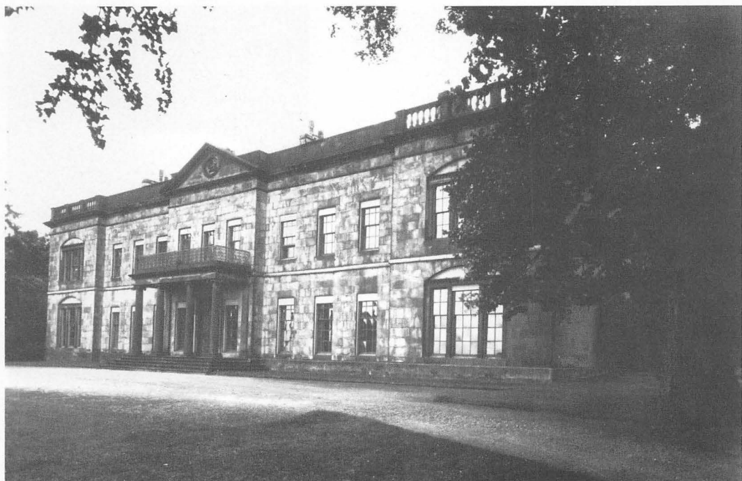
1. Shrigley Hall c. 1929.
