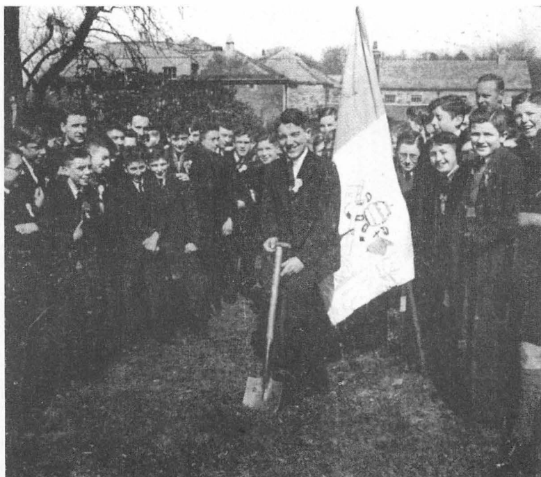
10. John Hoey Cuts the First Sod, 1 April 1934.
