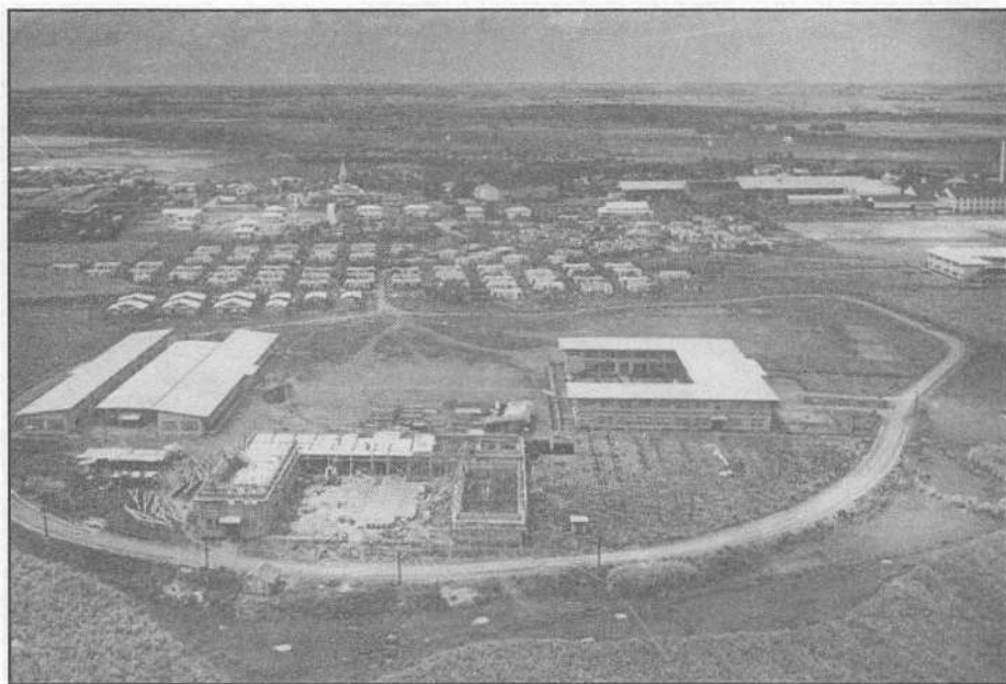
An aerial view of the on-going construction of the school of Don Bosco Victorias (1952), owned by Don Miguel Ossorio and the Victorias Milling Corporation.
